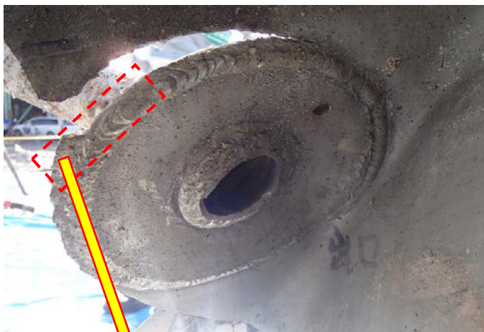
Outlet nozzle of cooling water water (observed from outside)
