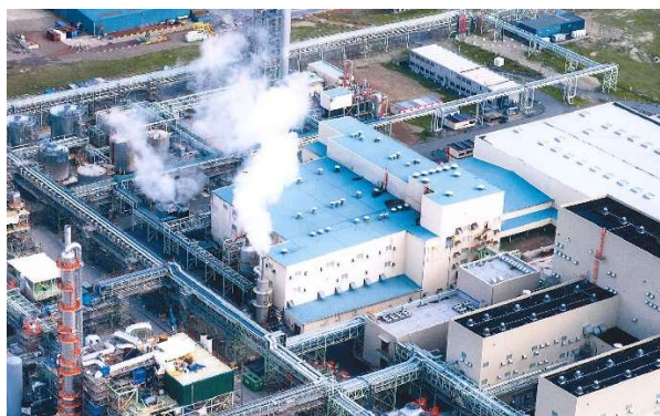
Pic.2 Aerial view of NSE site
