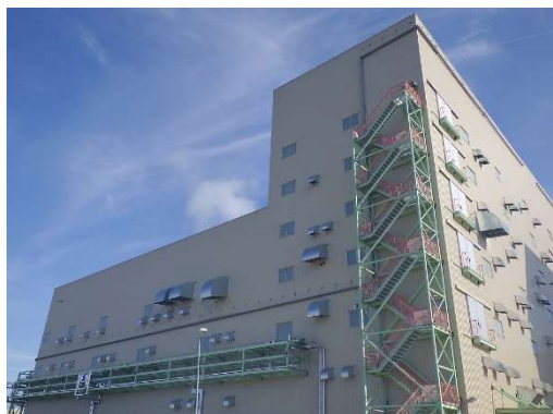
Pic.1 SAP Plant
