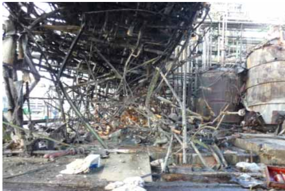
(Figure 4-8) Damages around V-3138
