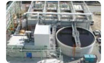
Activated sludge treatment system
