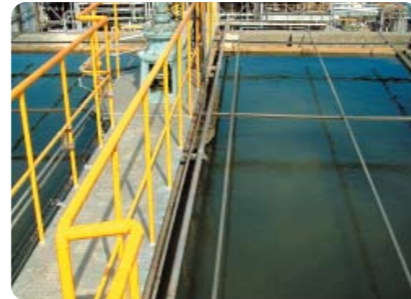
Activated sludge treatment system
