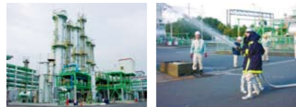
New glycol ethers plant (Kashima Plant)
