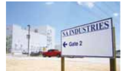
Superabsorbent polymer plant
