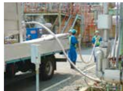
Emergency stabilizer injection drill
