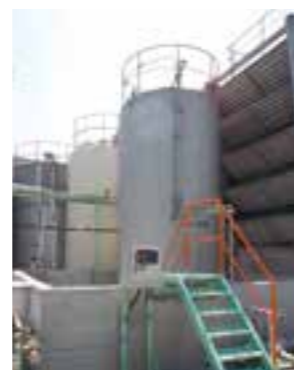
Installation of protective barrier for ammonia tank
