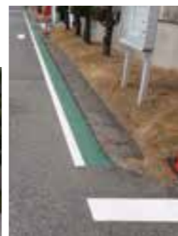
Re-painting of road markings
