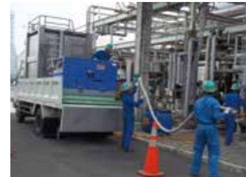
Training in emergency stabilizer injection drill
