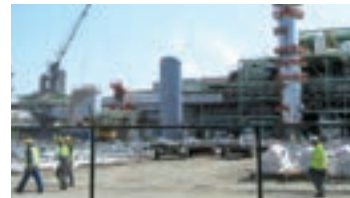
Acrylic Acid plant under construction
