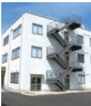
East side of new administration building
