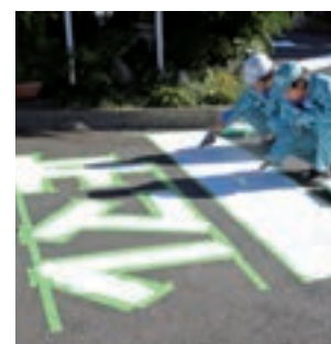
Road repairs under way
