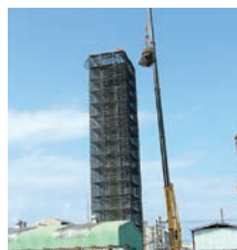
Smokestack disassembly
