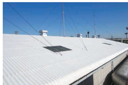
Thermal barrier-coated roof
