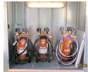
Mixed gas cylinders for injecting the polymerization inhibitor
