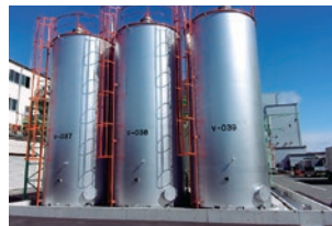
Tanks of caustic soda for cleaning and the dike
