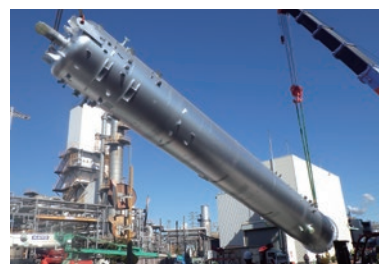
Absorption columns replacement at the Chidori Plant
