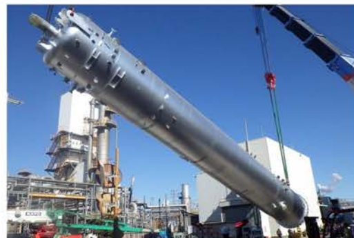
Absorption columns replacement at the Chidori Plant
