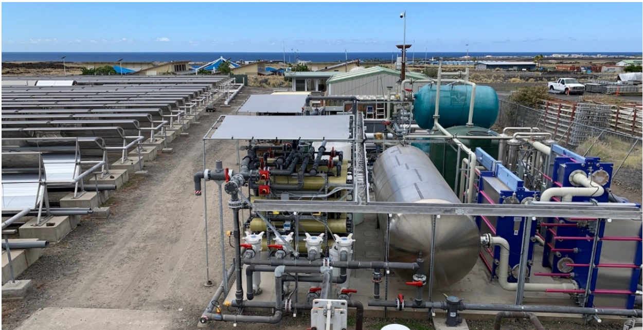
Photo 1 FO demonstration system for seawater desalination and water treatment. at a volume of 500 m 3 per day from seawater using the jointly developed draw solution on the islands of Hawaii by Trevi Systems
