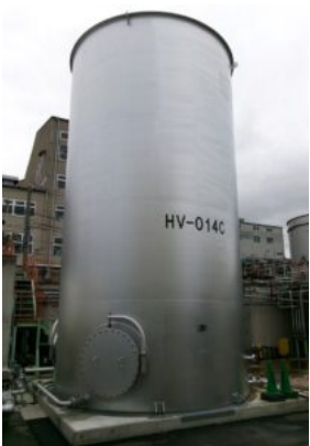
Newly installed raw water tank
