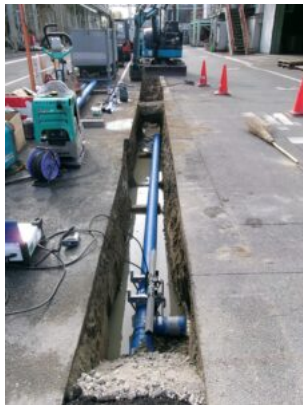
Renewal of fire hydrant piping
