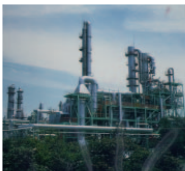
Chemicals Production Plant
