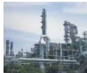
Chemicals Production Plant
