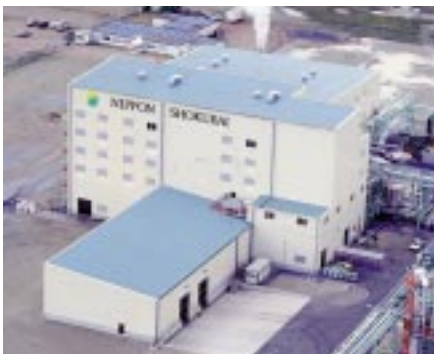
The new superabsorbent polymer plant.
