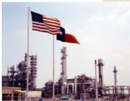
The near-to-completion acrylic acid plant (Annual production capacity, 120 thousand tons).
