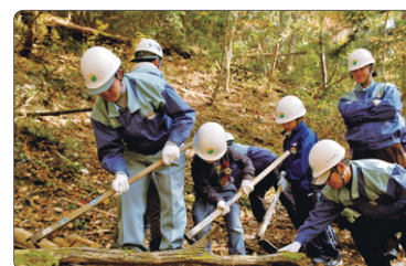
Nature trail construction
